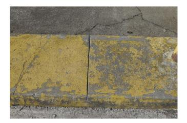
I expect the Town can remove these drive-thru caps by modestly deepening some of the saw cuts with an 18"+ concrete saw and adding the persuasion of a back hoe. The hope is that they would break off easily. It seems they were poured on the top of pre-existing concrete. I would want my existing drivethru overhang to remain undisturbed. I would supervise the work.
